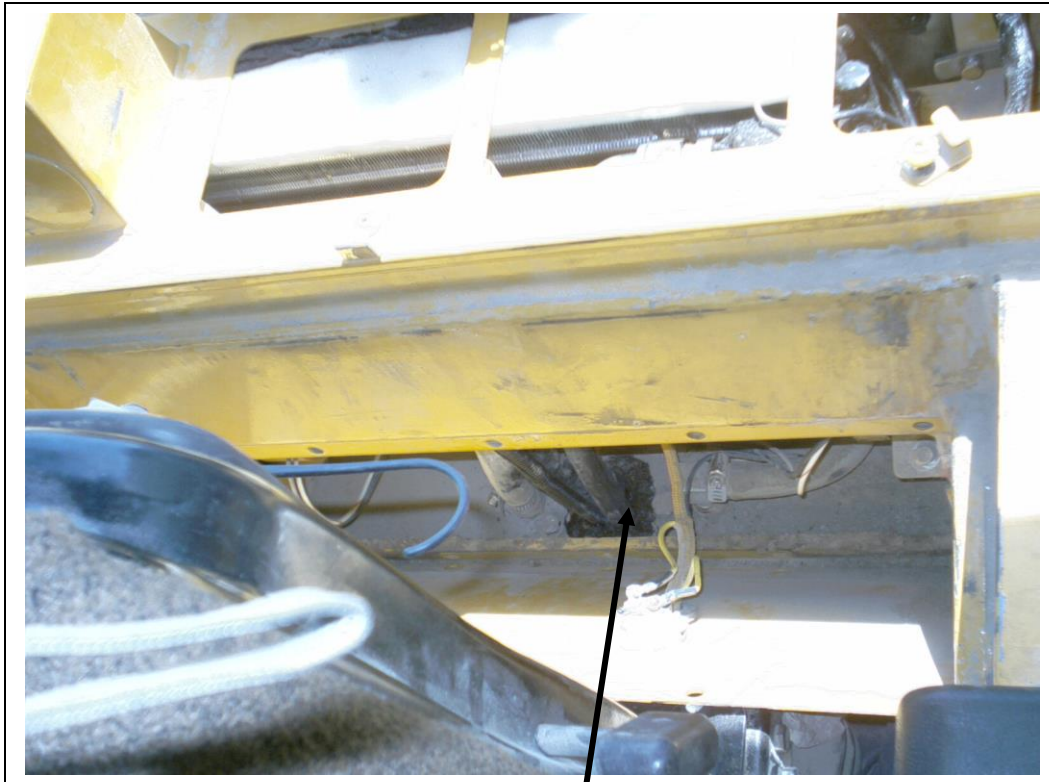
Seal opening with tar tape once the hoses are run into the cab
